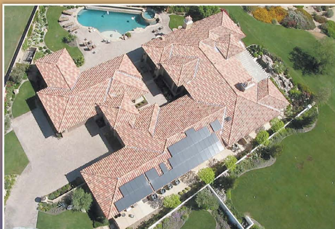
Toscana Country Club Solar Installation
