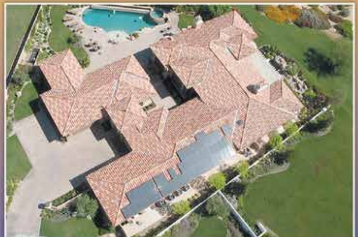
Toscana Country Club Solar Installation
