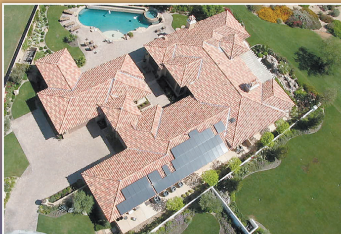
Toscana Country Club Solar Installation
