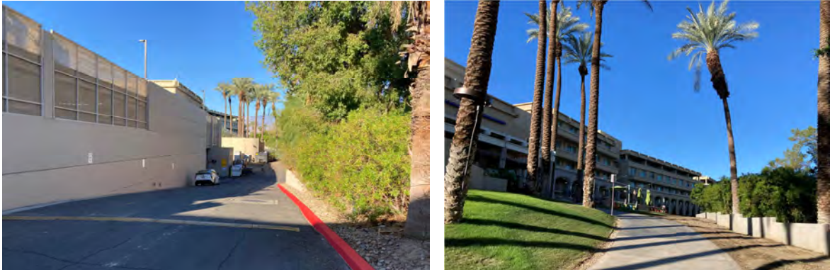
Shown here, the service road north of the parking structure. An actual path could be placed along the north side of this access road.
