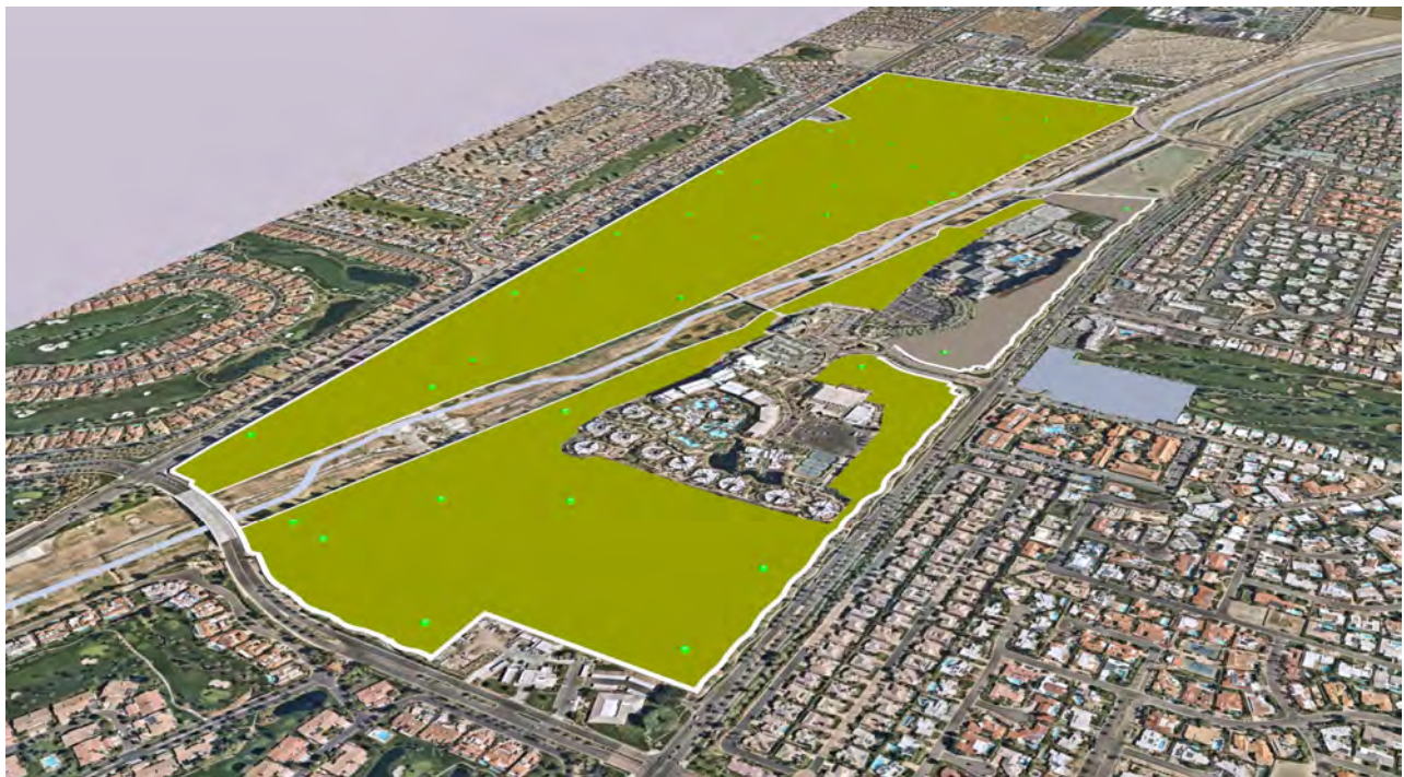
Shown above, an oblique view looking east over Indian Wells Golf Resort. The colored green area highlights the golf envelop that includes two golf courses and driving range. For exploring opportunities, the 17 th and 18 th holes of the Players course have been removed from the golf envelope.
