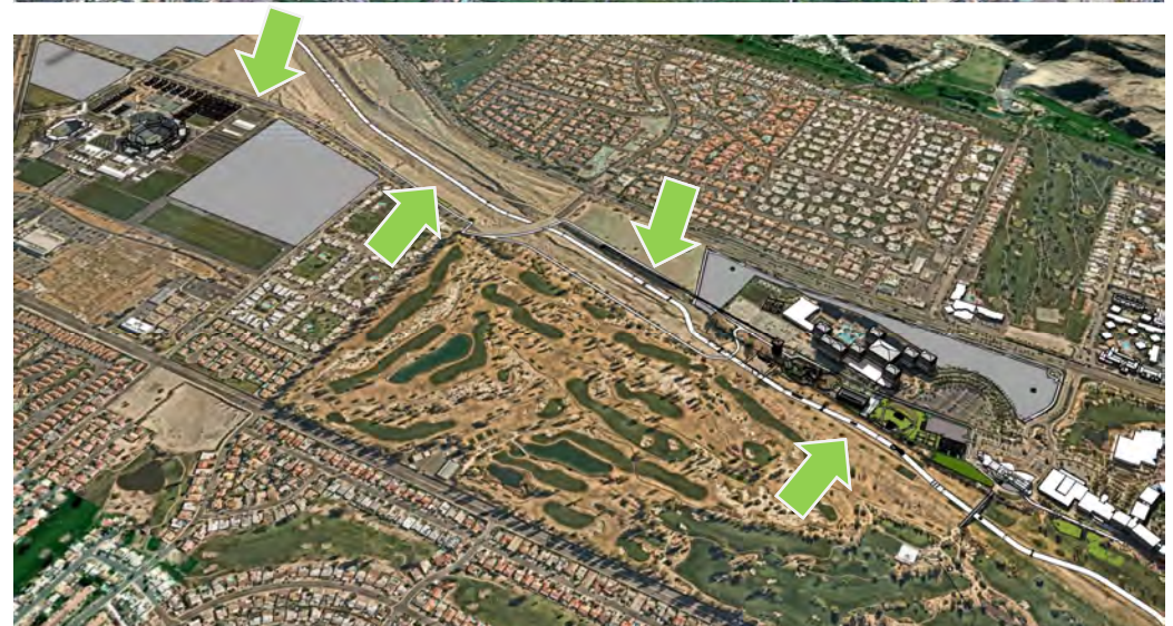
Shown at top above, IWGR and the Indian Wells Tennis Garden, along with select additional properties in the general area. Shown above, a linear multi-modal path along the Wash connecting the tennis and golf facilities, providing an amenity for residents and IWGR resort visitors.
